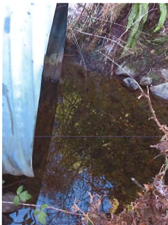
Photo 7. Culvert outlet of Hapifish Creek north of Peninsula Road showing no issues with fish passage.
